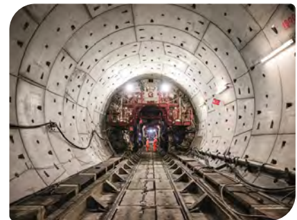
The Thames Tideway Tunnel under construction
