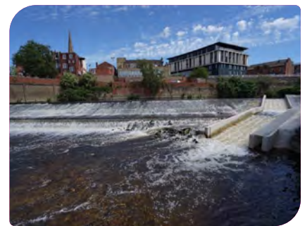
The new fish pass at Masbrough weir
