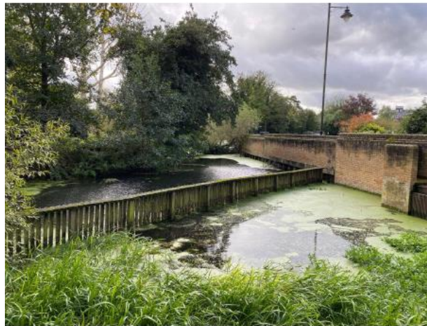
River Lark water levels lowered and edges of river realigned to increase biodiversity
