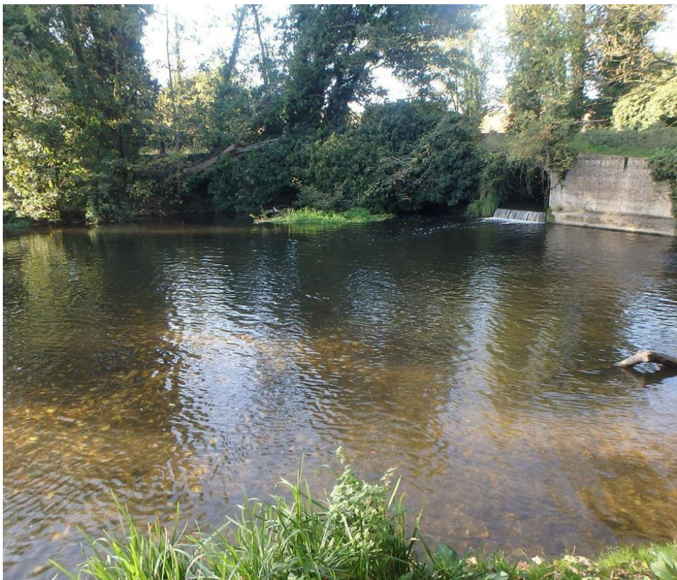
Fig 8. Gas Pool side sluices
