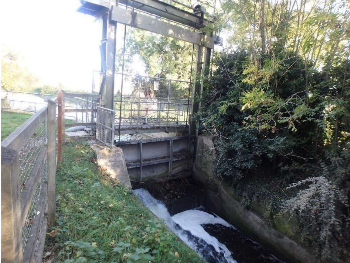
Fig 3. Gas Pool sluice, automated sluice gate and weir
