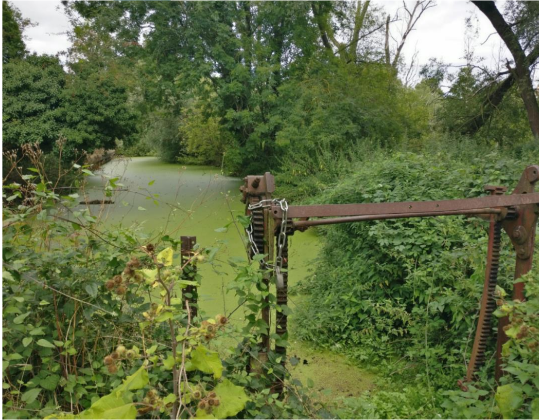
Fig 7. Back channel around Parkers Mill, structure that discharges in the Gas Pool
