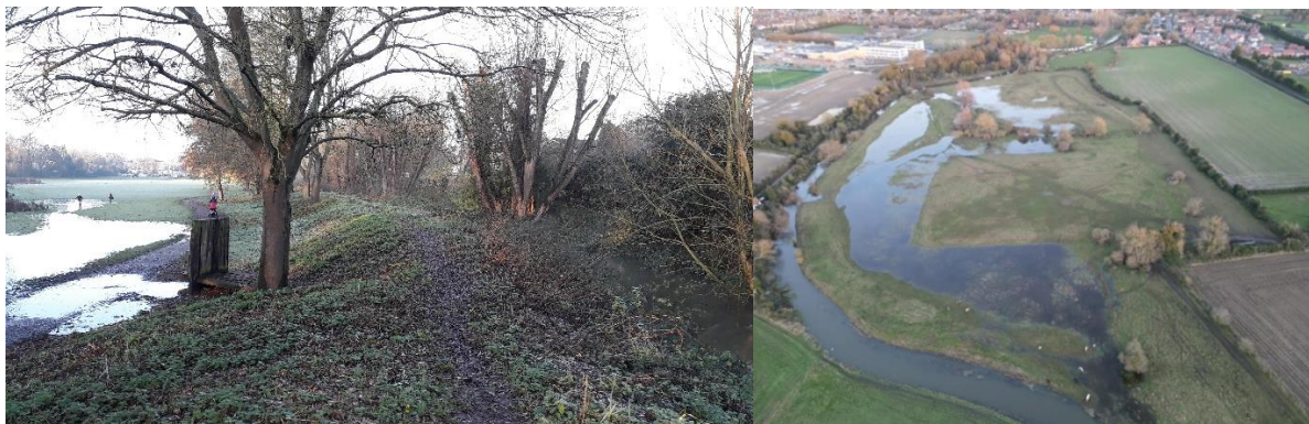
Photo 9: (Left) Embankment at Holywater meadows, BSE preventing floodwater from draining back into river Linnet/
